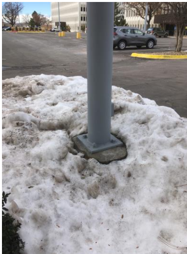
Figure 6: Pole number 12 with large pile of snow plowed around the base.
