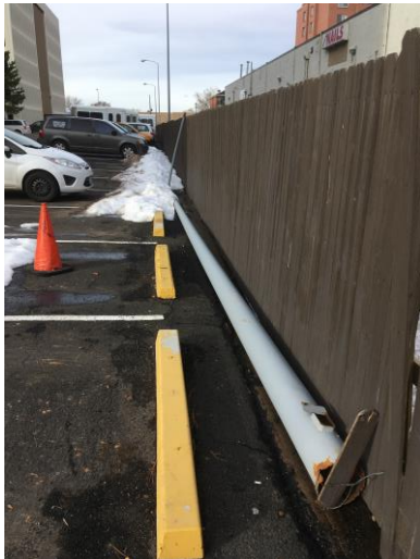
Figure 1: Downed light pole on NE corner of the property.
